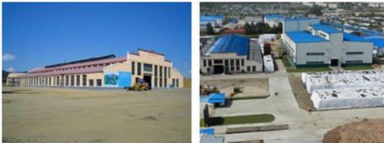
Facilities of Tahe Biopower Plant
