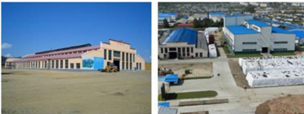
Facilities of Tahe Biopower Plant
