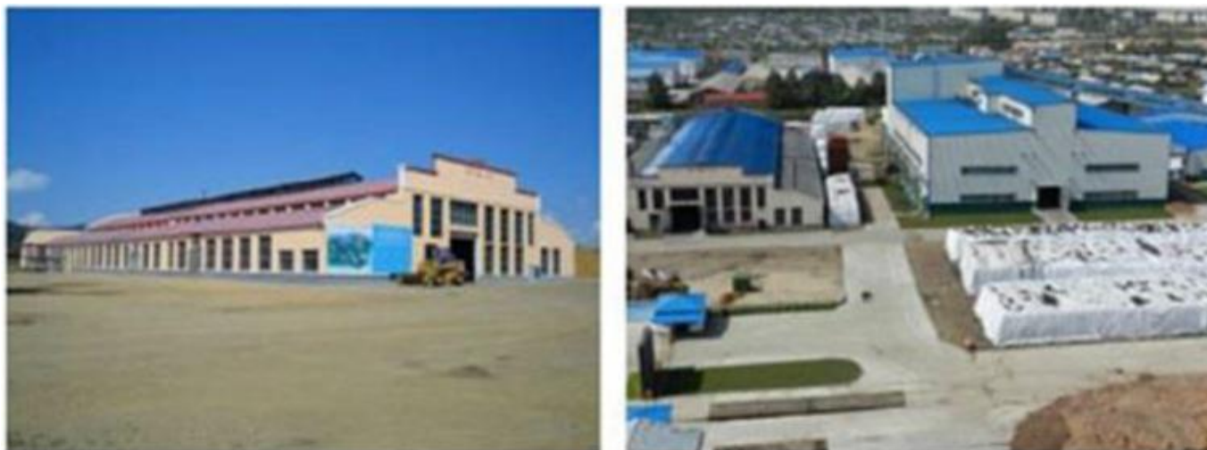
Facilities of Tahe Biopower Plant
