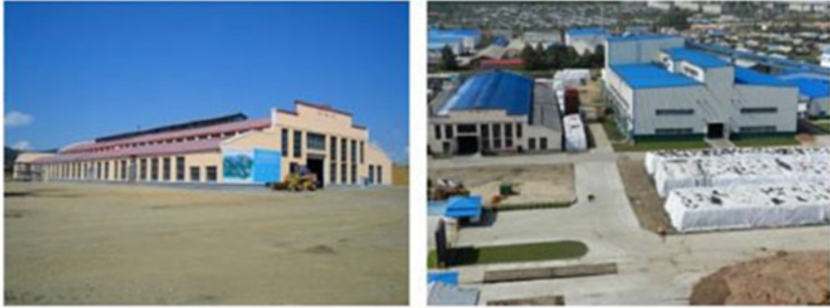
Facilities of Tahe Biopower Plant
