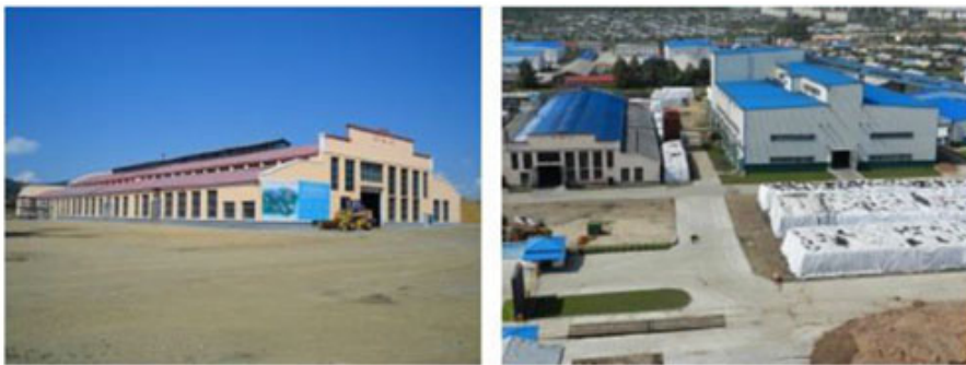
Facilities of Tahe Biopower Plant
