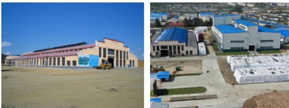
Facilities of Tahe Biopower Plant
