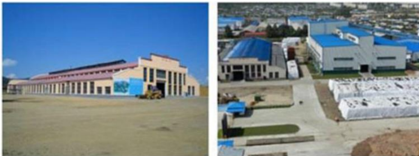
Facilities of Tahe Biopower Plant
