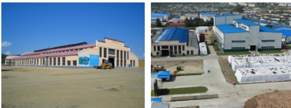
Facilities of Tahe Biopower Plant
