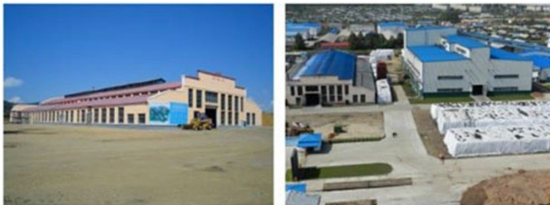
Facilities of Tahe Biopower Plant
